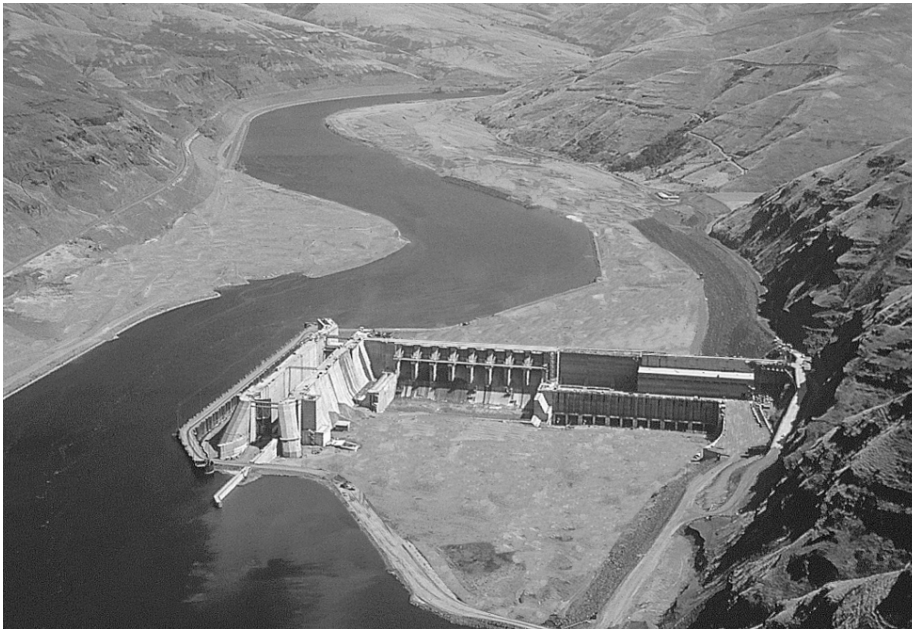
Figure 5.15-2. Site Condition During Construction of Lower Granite Dam That May Be Similar to the Breached Condition
