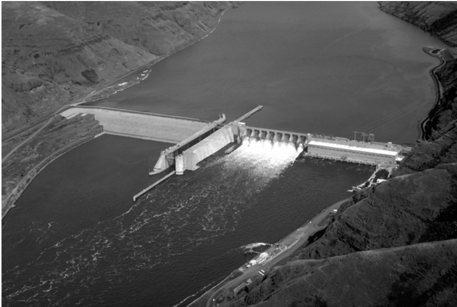
Figure 5.15-1. Current Photograph of the Lower Granite Dam Representative of the First Three Alternatives
